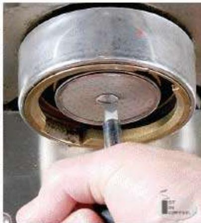
**Removing this screw allows the shower screen and the shower head to be removed for cleaning**
